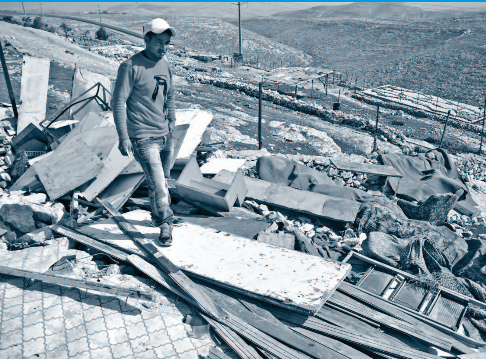
Jabril Jahalin stands at the site of his demolished home
